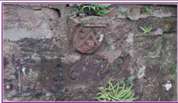
Architectural skewputt and lintel dated 1629 outside the main entrance Alyth
