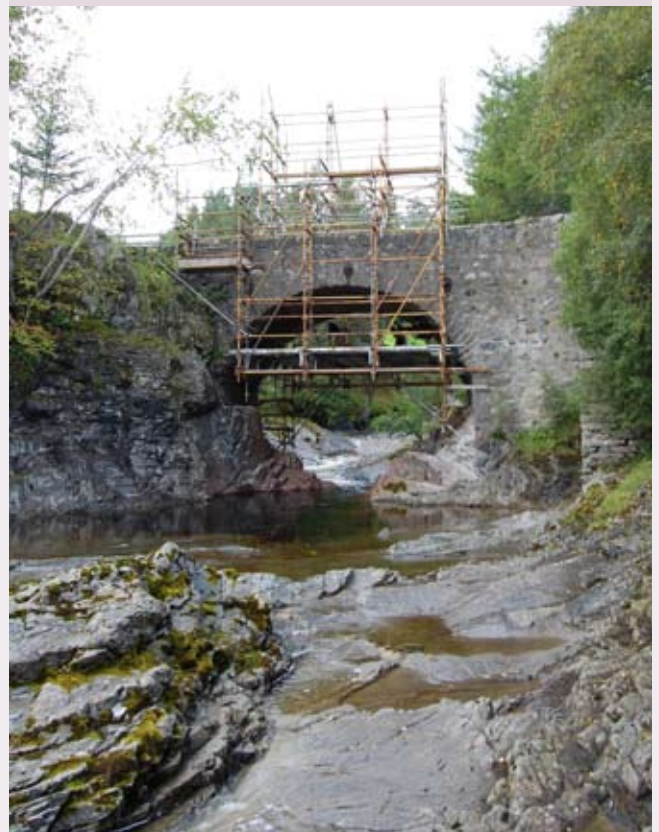
The innovative scaffold carriageway at Dalnamein.
