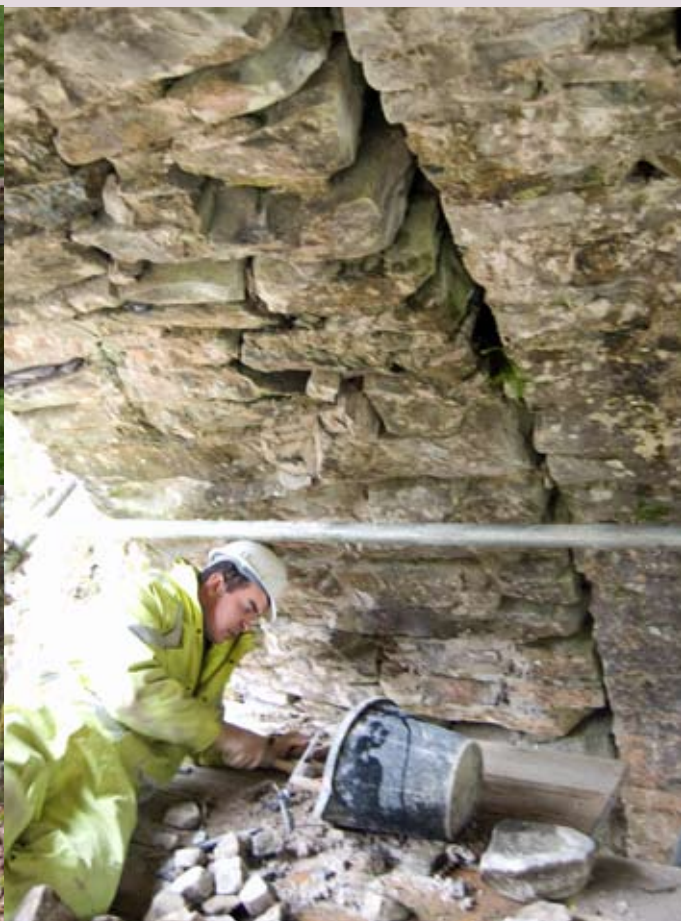
Pinning and re-pointing the soffit of Dalnamein Bridge, on the A9 near Calvine.
