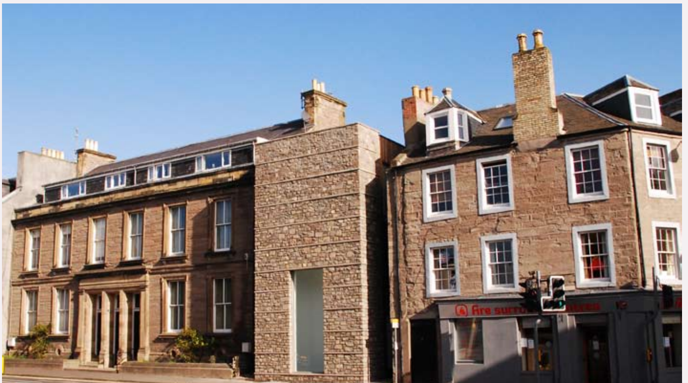
5a Melville Street, Perth (© Fergus Purdie Architect).
