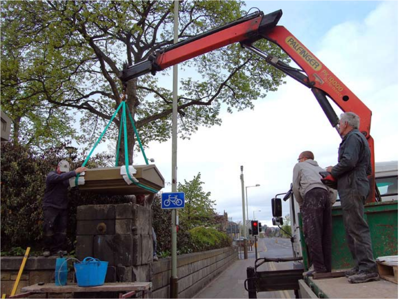
Replacing the stone pier caps at the AK Bell Library, Perth.
