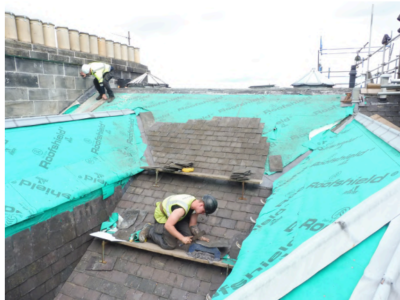
1 King's Place - full comprehensive building repair including re-slating and re-pointing
