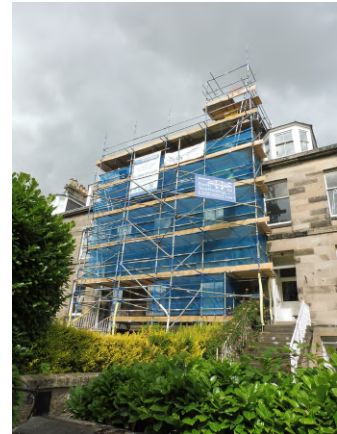
1 King's Place - full comprehensive building repair including re-slating and re-pointing
