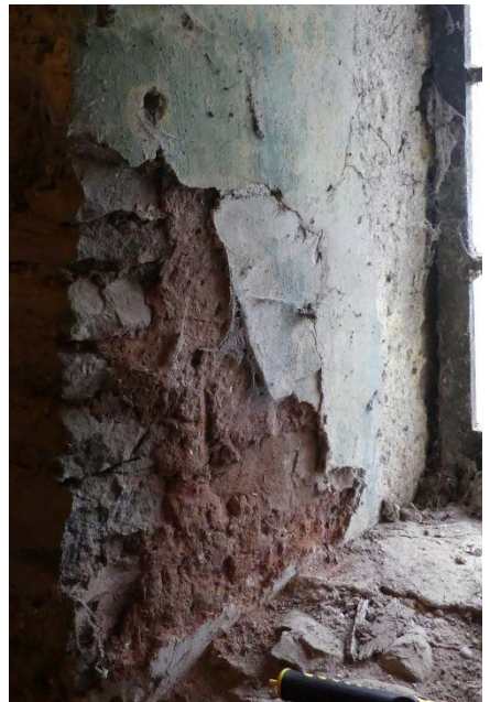
Earth plaster base coat below a lime top coat at Craigdallie .
