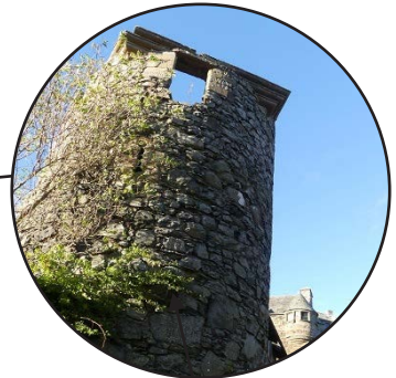
Elcho Castle is a good example of a high status building, where clay was used in the walls and floor of a corner tower around 1560.
