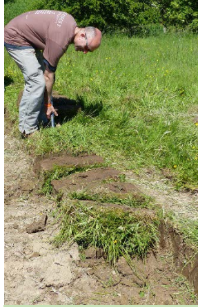
Cutting turf blocks.
