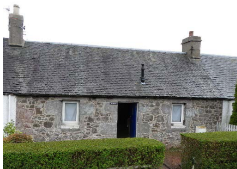
Typical clay mortared & slate roofed house, Longforgan, built around 1800.
