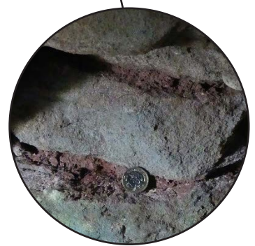
The 15 th century Carmelite Friary on Whitefriars Street in Perth was located just outside the medieval city walls. The excavated walls are clay bonded, probably to create a damp-proof foundation for lime mortared walls above.
