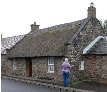
Typical clay mortared and thatched house, Longforgan, built around 1800.
