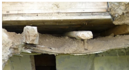
Earth deafening infill at Horn Farmhouse.
