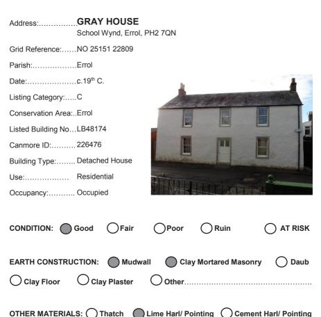
**ASSESSMENT:** Gray House is a mudwall house, with numerous alterations, mainly in clay mortared masonry and brick. It underwent extensive repairs as part of the TLP, and this is recorded in a HES Good Repair Guide. Remnants of broom thatch in the roof space were found although, like all Errol buildings, it is now slated. The south gable was faced with concrete block after demolition of the neighbouring building, which was semi-detached, leaving this one alone.
